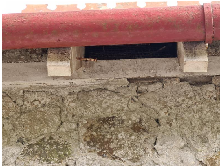
Photograph 2: Eaves level potential access point
