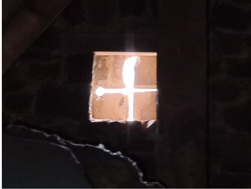
Photograph 4: Cross shaped unmeshed ventilation in the gable walls viewed from inside the roof space (also shown on Photograph 1 from the outside)
