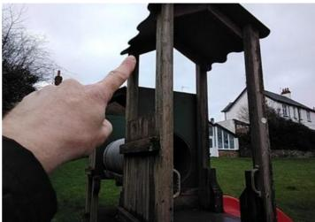
**Finding:** There is or are fixings missing on the roof panels
