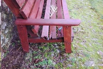
**Finding:** There are areas or parts of the timber on the structure that have rotted through structural integrity of the slats cannot be determined
