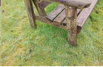
Finding: The bench/es is/are not securely fixed to the surface and there is some possibility of the item/s tipping or rolling over
