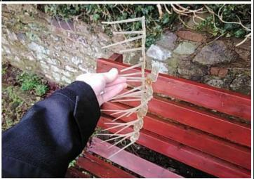
**Finding:** There are hard needle-like plastic bird deterrent strips on the crossbar. We don't recommend the use of these devices. Two sections had fallen from the crossbar at the time of the inspection
