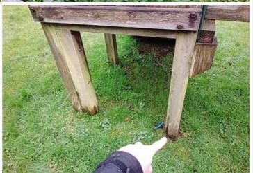
Finding: There are areas or parts of the timber post on the Action: Replace all affected timbers climb panel tower that have rotted
