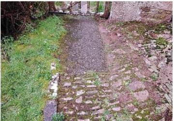
**Finding:** There is algae, silt or moss growth on the footpath **Action:** Clean and treat appropriately surface resulting in slippery conditions
