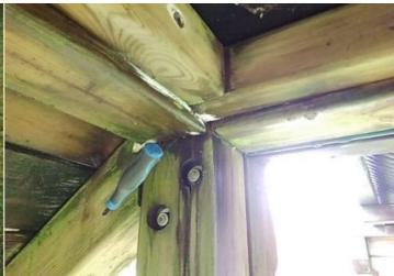
**Finding:** There are areas or parts of the timber post that have rotted at the base and around the area where the platform is mounted
