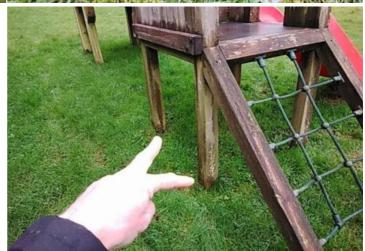
**Finding:** There are areas or parts of two timber posts on the **Action:** Replace all affected timbers slide tower that have rotted
