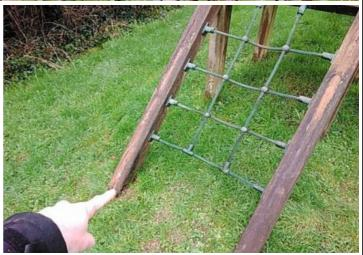
**Finding:** There are areas or parts of the timber net frame on **Action:** Replace all affected timbers the structure that have rotted and sheared
