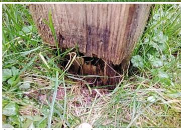
**Finding:** NOTE - A post has previously rotted and an additional post has been installed to stabilize the structure
